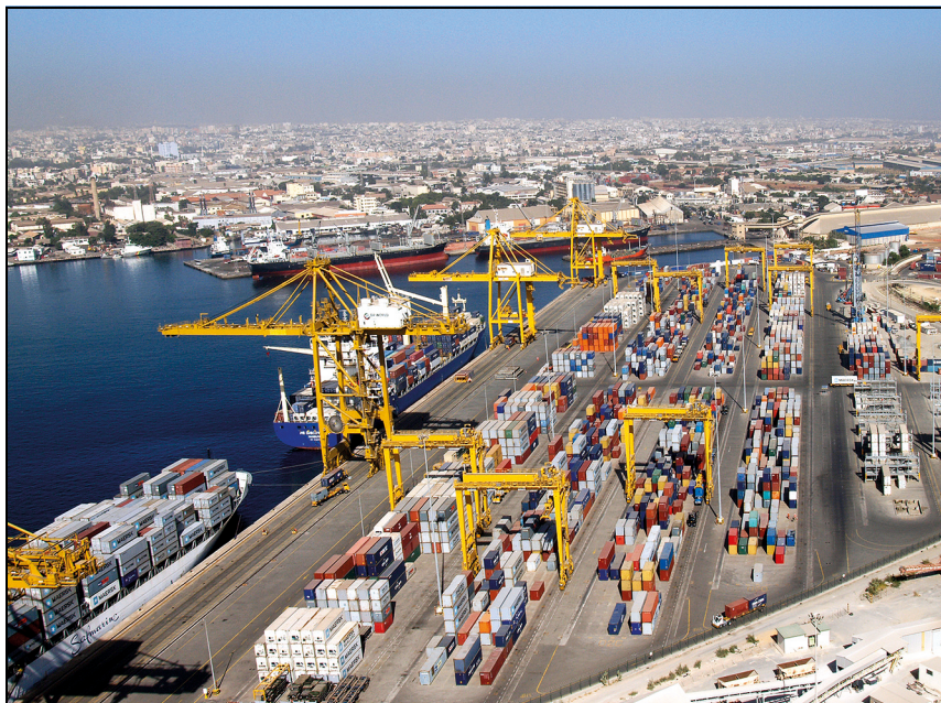
Figure 2.1 Senegal. Container terminal in Dakar.
