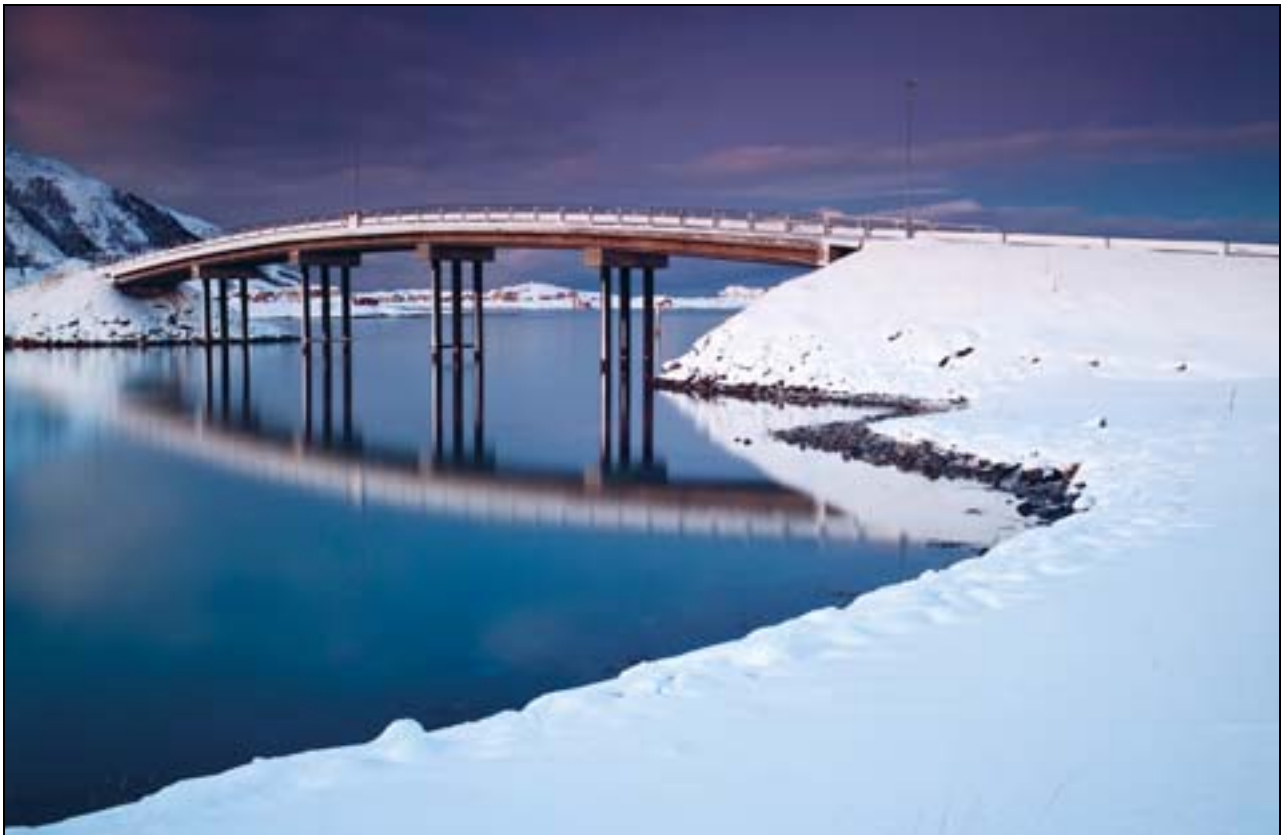
Figure 2.1 Bridge between Sommarøy and Hillesøy in Troms.
