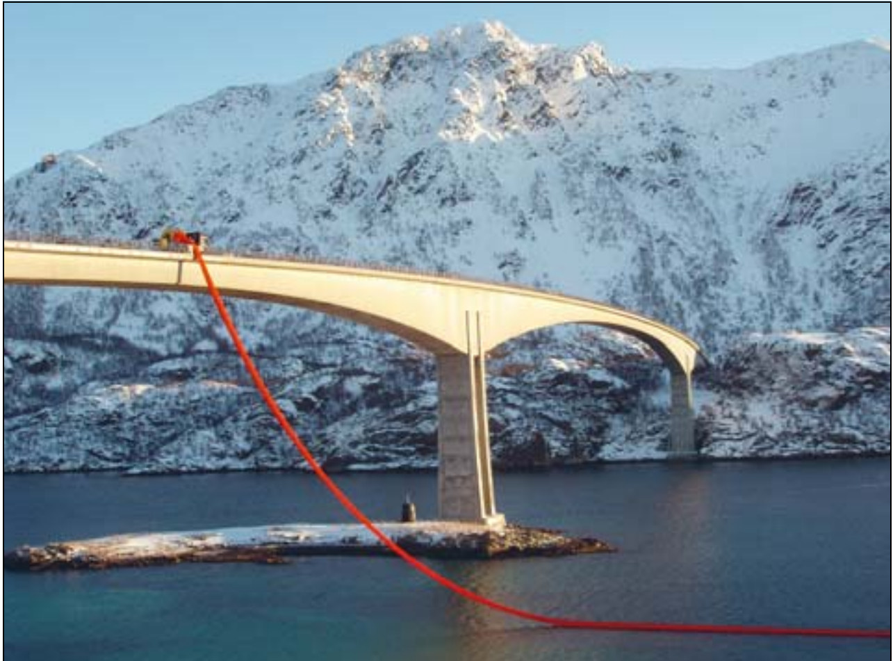
Figure 10.2 Testing an oil boom from the bridge across Raftsund in Nordland county.
