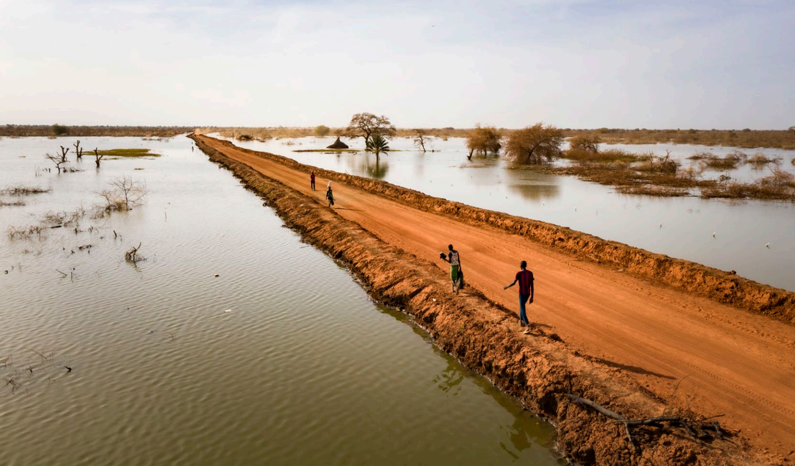
Thousands of people are permanently displaced after years of flooding in Bentiu, South Sudan. This road is protected by dykes and cuts through the floodwater. The road stretches all the way to the horizon, near Bentiu.
