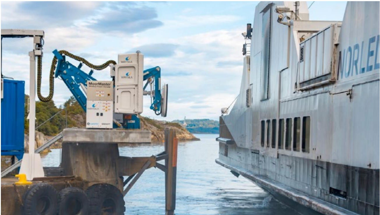
In a world first, an automatic wireless induction charging system and automated mooring technology have been successfully tested for the car ferry MF Folgefonn.
