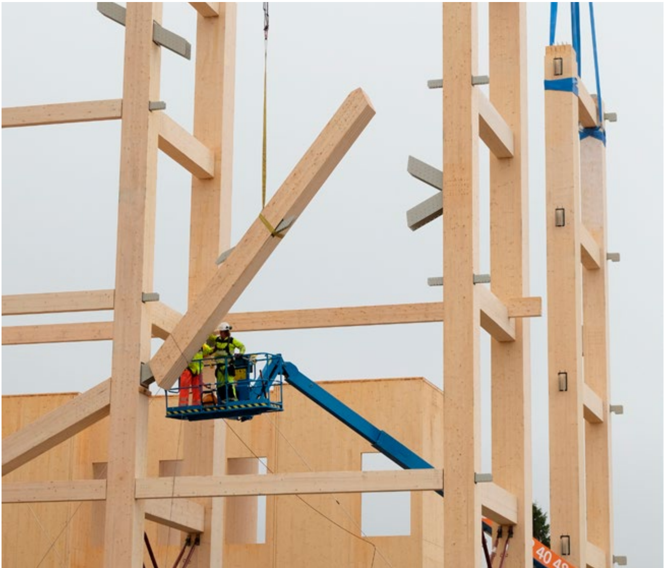
'Mjøstårnet' (the Mjøsa tower) is under construction in Norway, and at 81 metres will be the world's tallest wooden building when it is completed in February 2019. Using more wood in buildings can be a way of increasing the carbon stock in long-life wooden structures.
