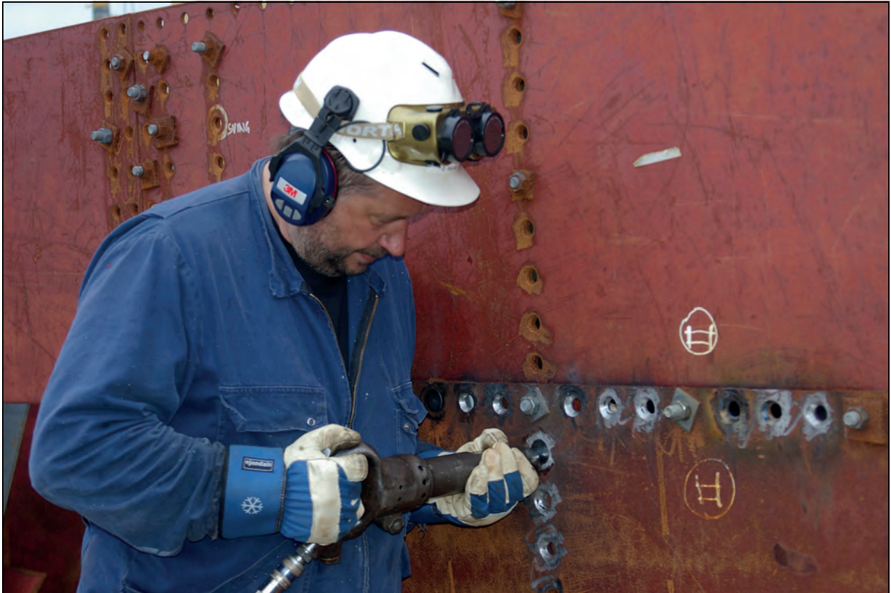
Figure 8.10 Riveting a steel vessel at Bredalsholmen Shipyard and Preservation Centre (BDF).
