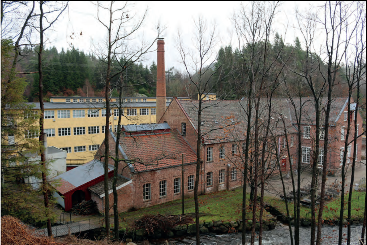
Figure 4.4 The wool mill Sjølingstad Uldvarefabrik was protected in 2019.
