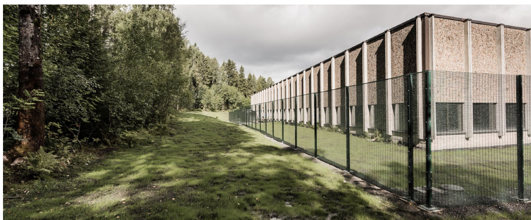
One of Basefarm's two data centres outside Oslo
